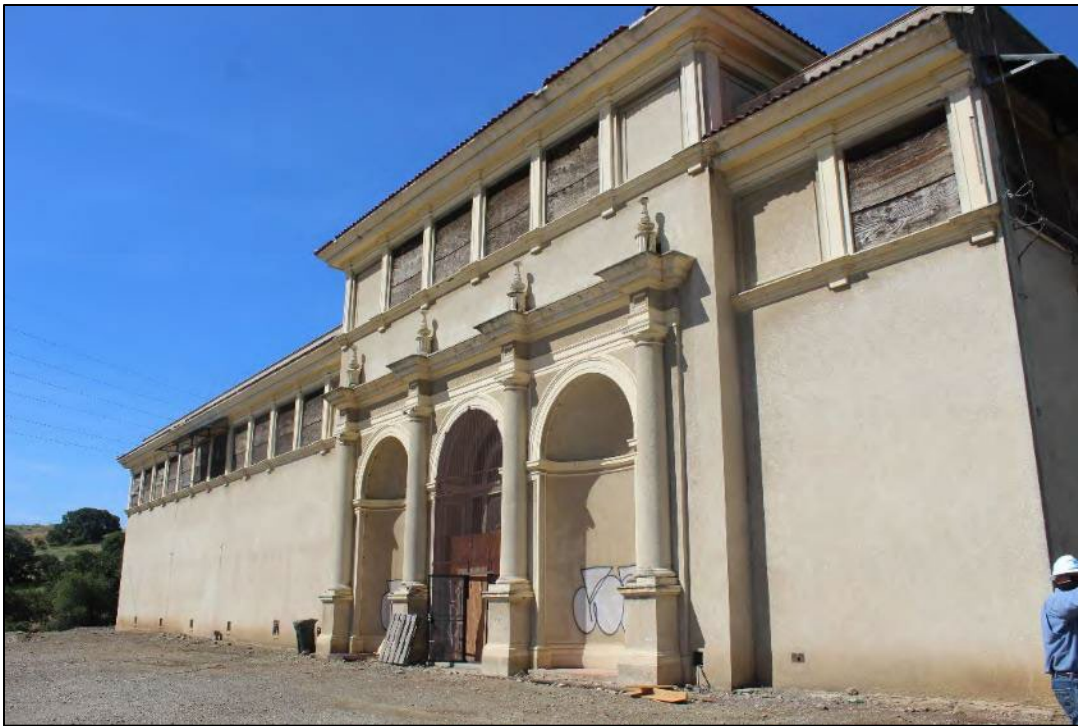
Photograph 5: East elevation of the Cordelia Substation, camera facing southwest. April 29, 2021.
