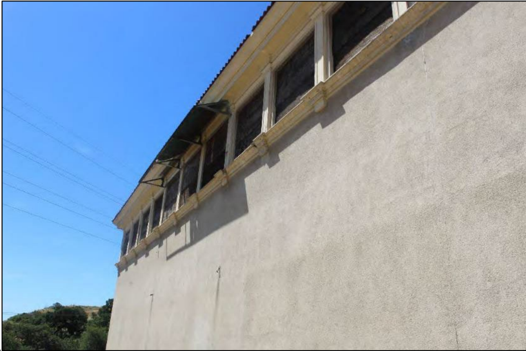
Photograph 11: Windows on the east elevation, camera facing southwest. April 29, 2021.
