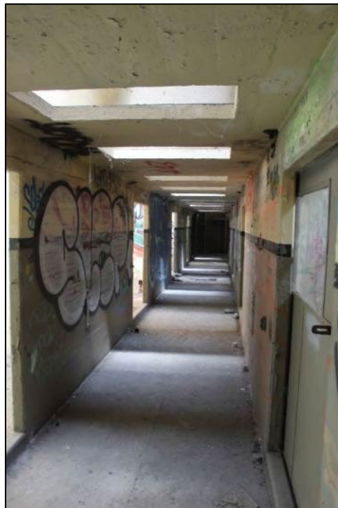
Photograph 14: Hallway leading to bus cells, camera facing south. April 29, 2021.
