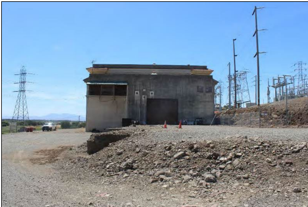
Photograph 2: North elevation of the Cordelia Substation showing terraces and separation of control building and active switchyard, camera facing south. April 29, 2021.
