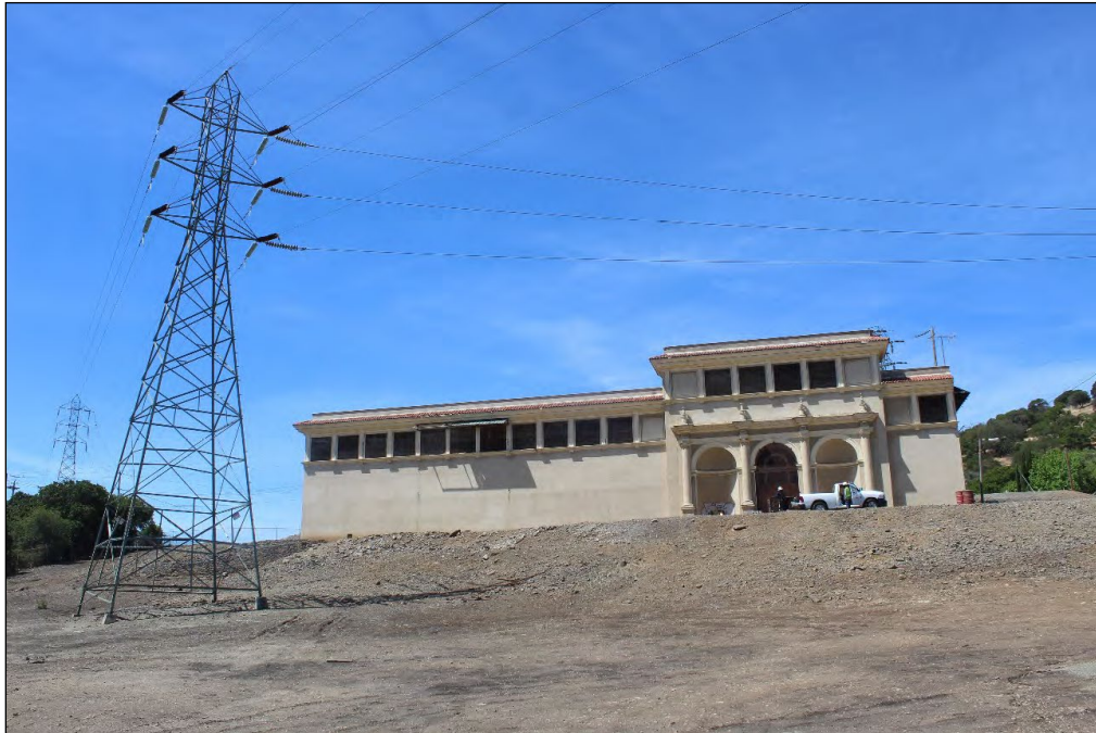
Photograph 1: The Cordelia Substation, camera facing west. April 29, 2021.
