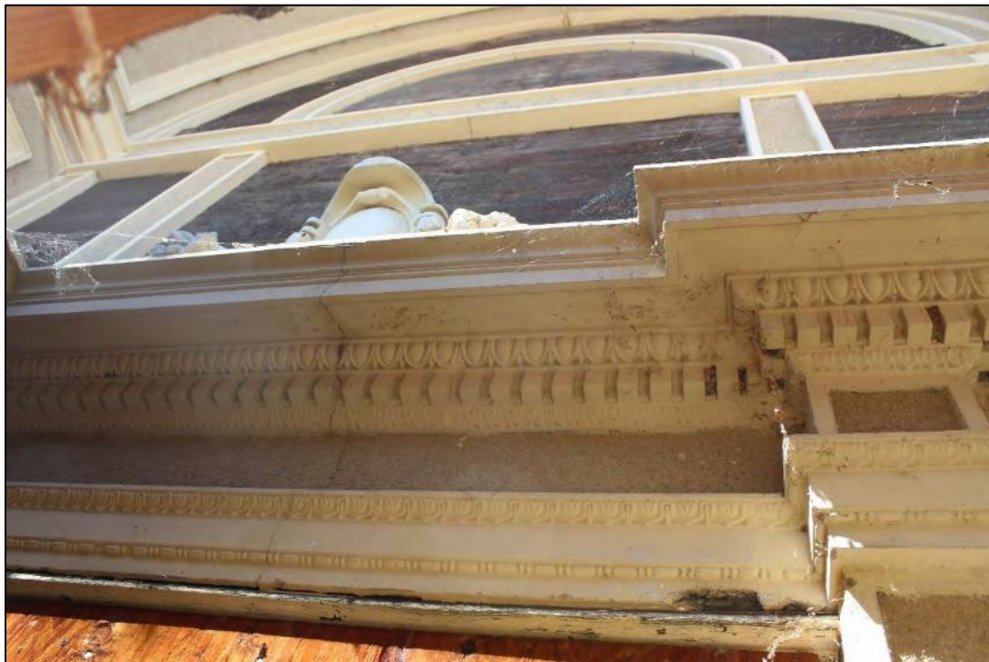
Photograph 10: Concrete cartouche on the entryway cornice, camera facing southwest. April 29, 2021.
